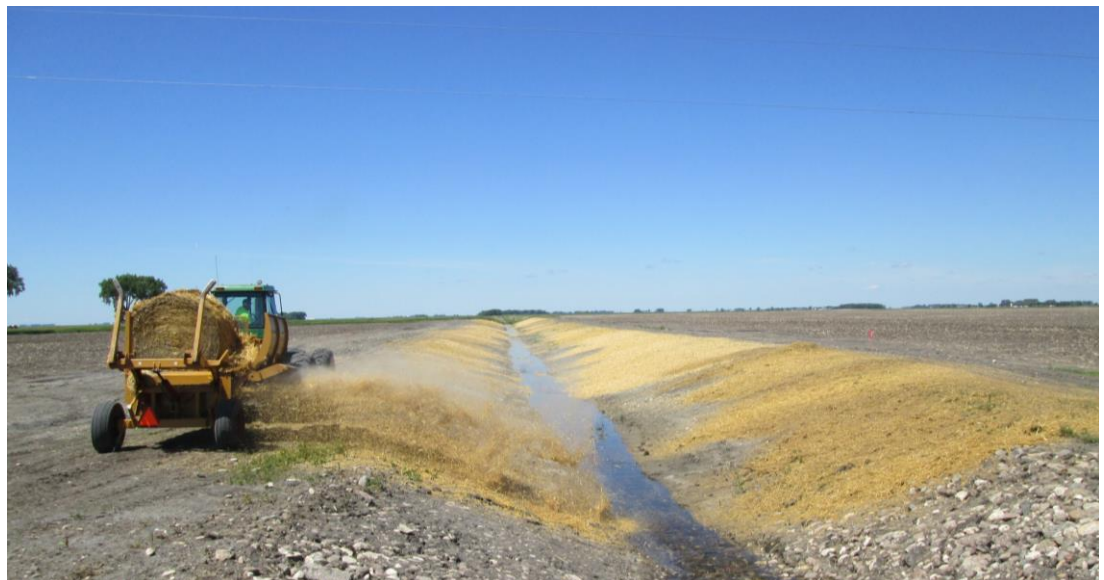
Mulching at the project site. Project completed June 2020.
